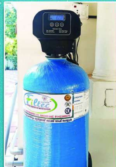
W.T.P. 1000 lph iron removal Automatic plant
